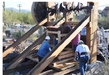
Installation of ore feeder
